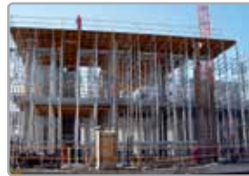
CONSTRUCTION Formwork and scaffolding
